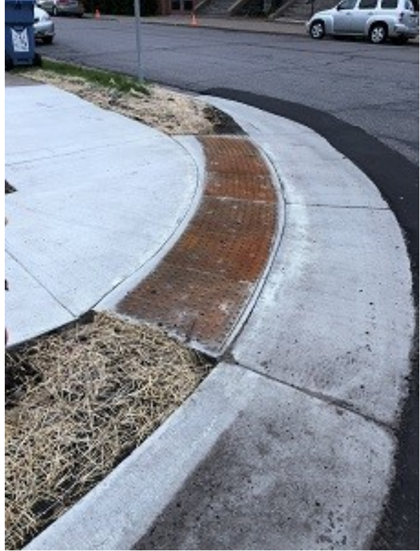
Photo of the new ADA sidewalks on Monroe & 13th
